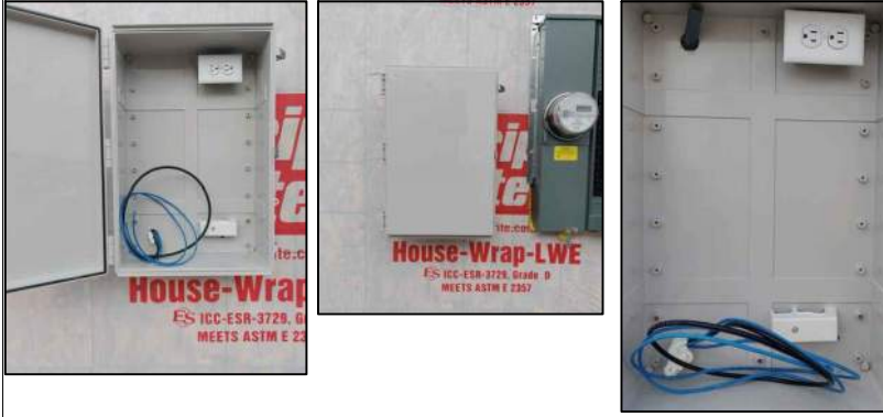
EXAMPLE 1 OF EXTERIOR COMMUNICATION WALL MOUNT
