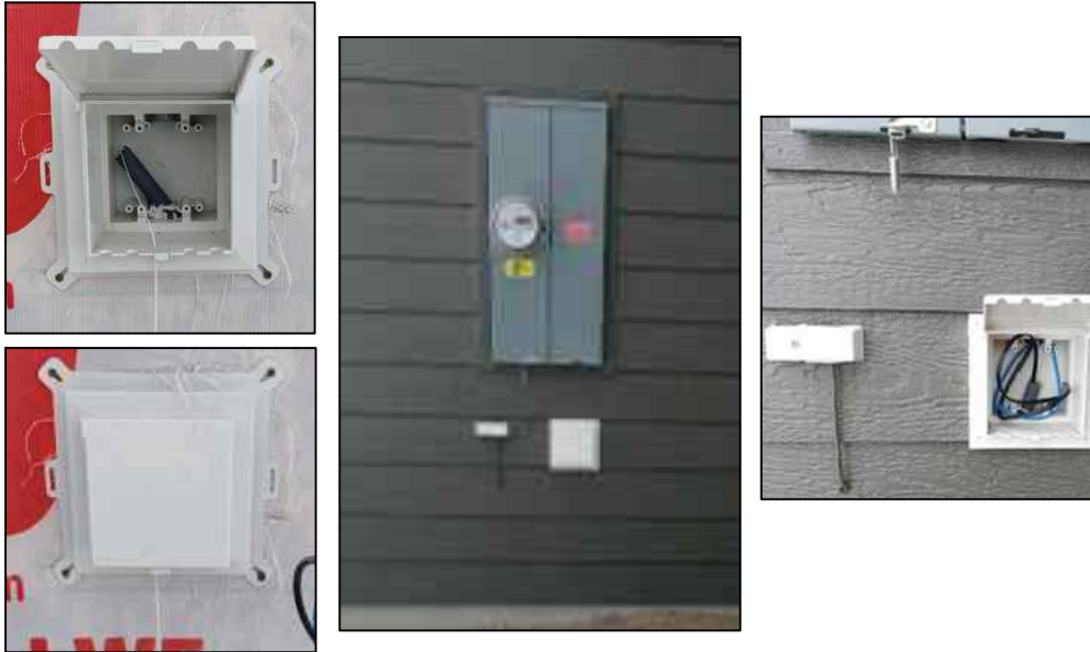
PREFERRED METHOD OF FIBER INSTALLATION
