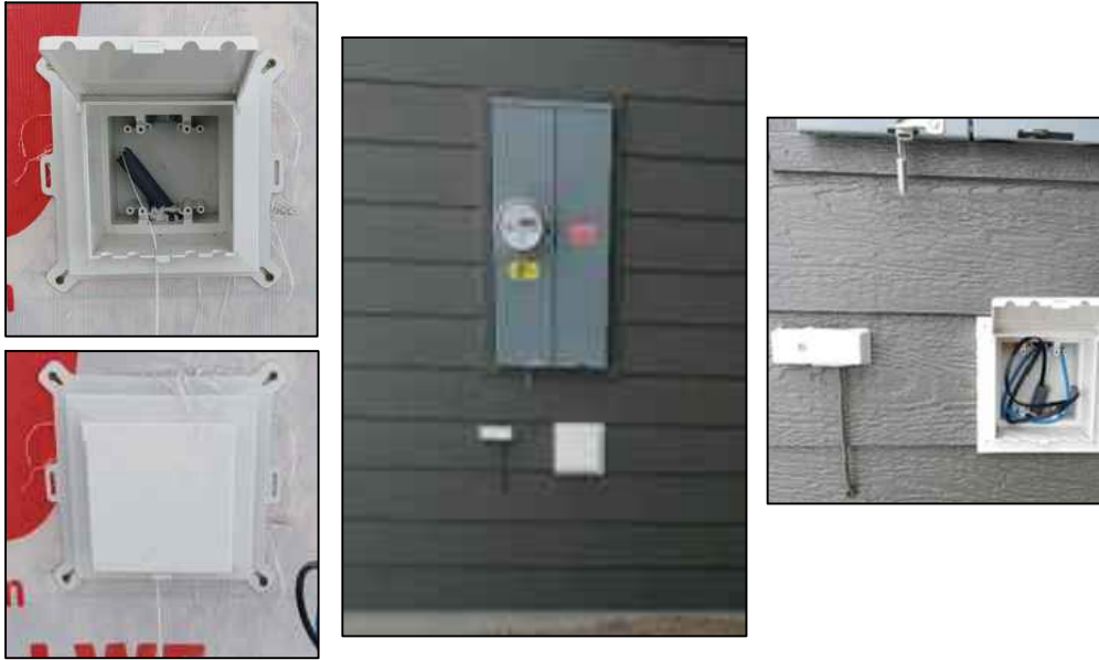
PREFERRED METHOD OF FIBER INSTALLATION
