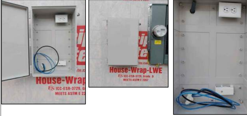
EXAMPLE 1 OF EXTERIOR COMMUNICATION WALL MOUNT
