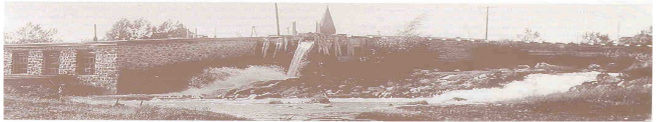
The original 1900 power plant generated electricity from the water tumbling out of an irrigation ditch.
