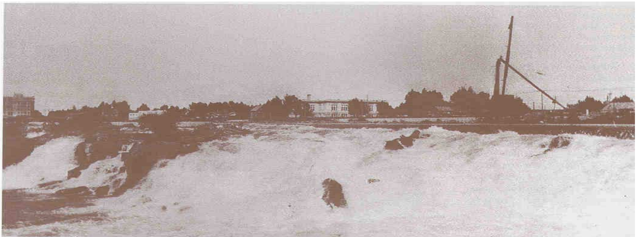
THE DERRICK IN THE MIDDLE OF THE FALLS WAS USED IN THE 1920S AND 1930S TO REMOVE LARGE ROCKS BLASTED LOOSE FROM THE MAIN CHANNEL OF THE SNAKE RIVER, INCREASING FLOW THROUGH THE CITY PLANT.
