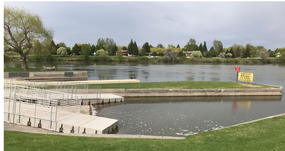
South Tourist Park Boat Launch, Lower Plant
